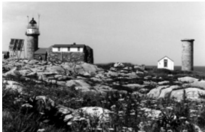
The Coast Guard disassembled most of the buildings from the original Light Keeper community. Today, structures include the Lighthouse, Boat House, Audubon House, and two light towers.
